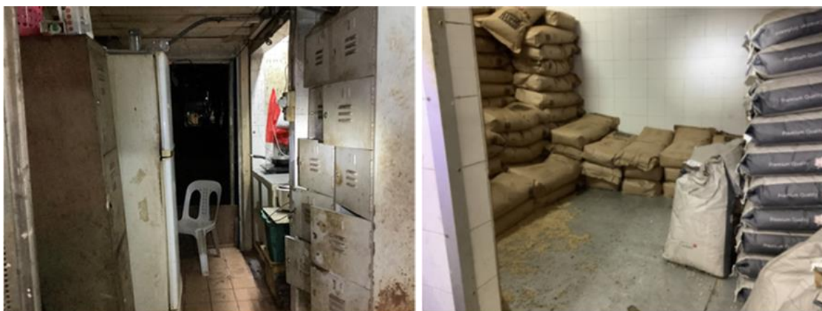
The premises was found to be poorly maintained. (Photos: SFA)
