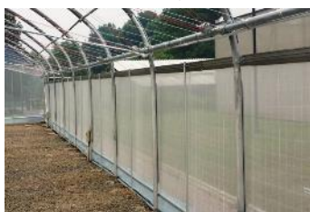
Perforated side netting as pest barrier
