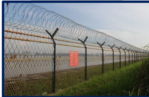
Fencing at Punggol Barat
